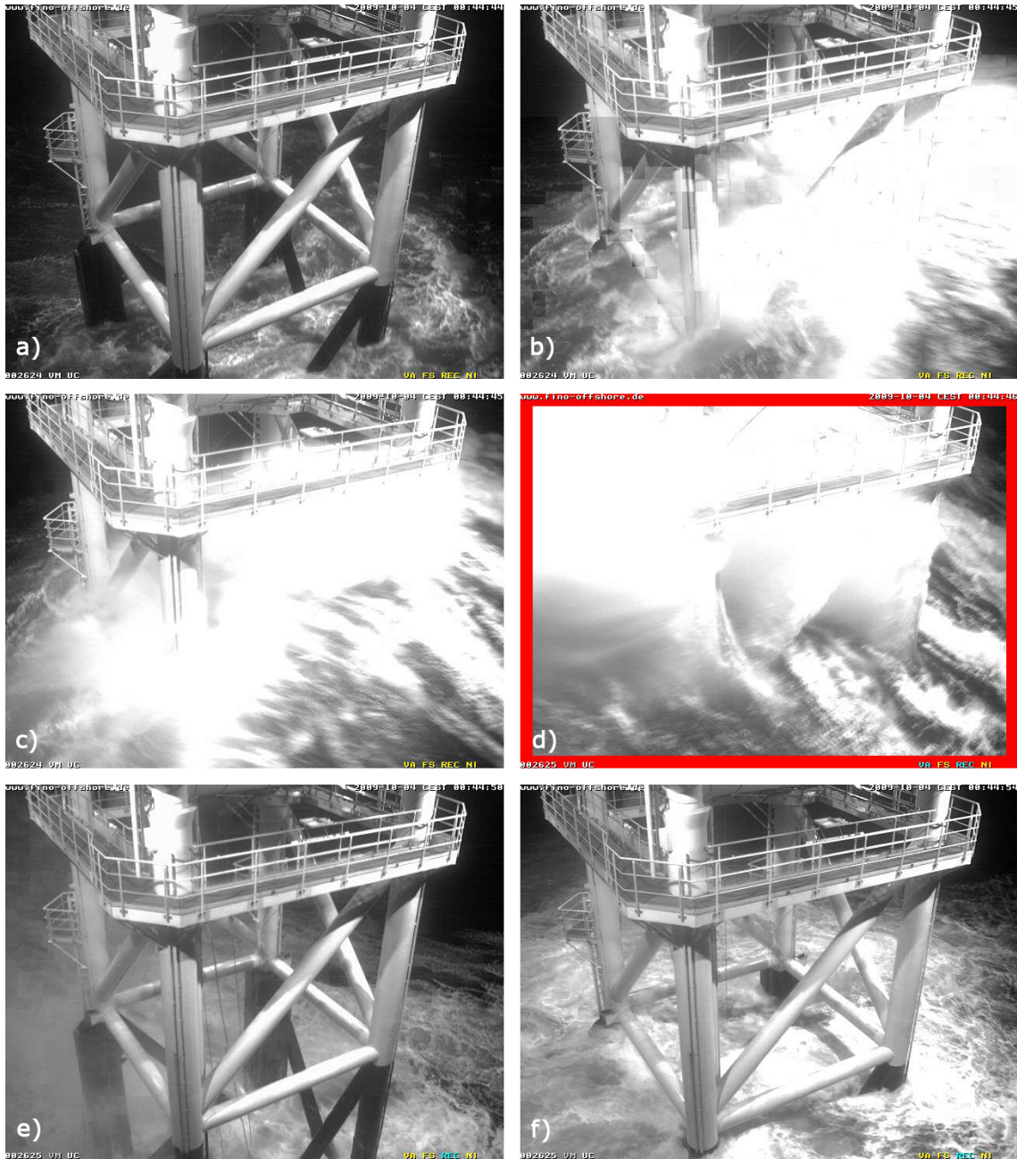
Figure 1.6: Snapshots of an approximately 15m high breaking wave with a crest to crest period of 9s captured at FINO I on the 4th of October 2009. The time shifts of the frames in relation to snapshot a) are +1.402s (b), +1.682s (c), +2.383s (d), +6.2s (e, subsequent trough), +10.597s (f, subsequent crest). , For orientation, the center to center spacing of the main columns is 7.5m and the hand rail is 15m above LAT.
