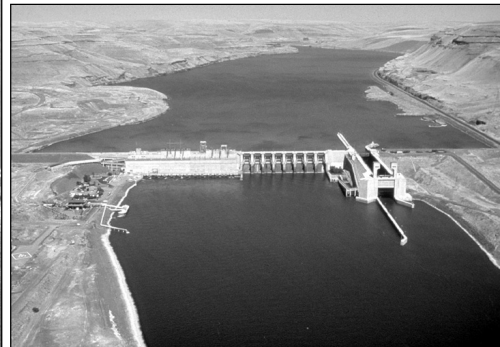
Tows on Columbia/Snake system in Pacific Northwest use unique locks with lifts over 30 meters. Tows can draft 4.3 m.
